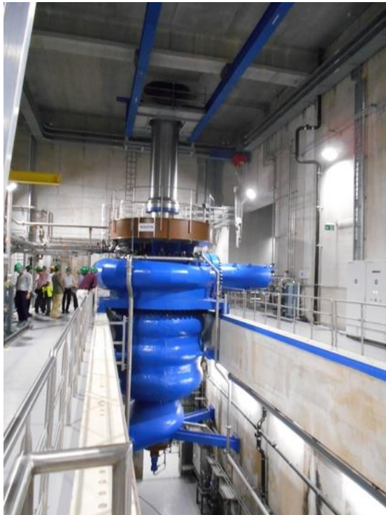
Reverse pump at the Veytaux pump storage installation
